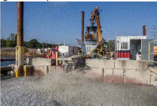
Figure 13: Broadcast Capping System
