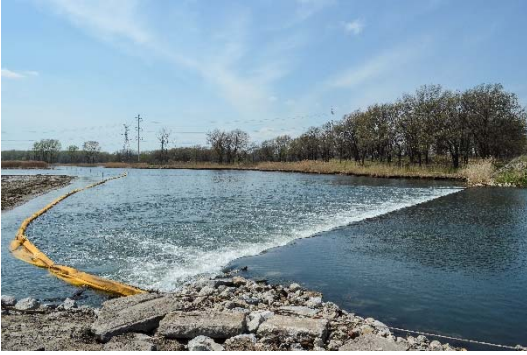
Figure 1: Sheet pile barrier wall
