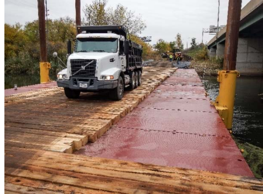
Figure 12: Temporary floating bridge
