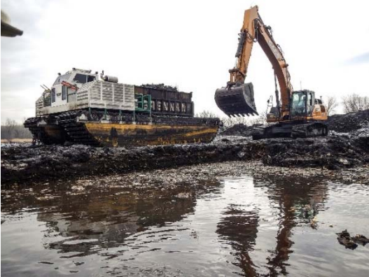
Figure 11: Amphibious excavation of wetlands
