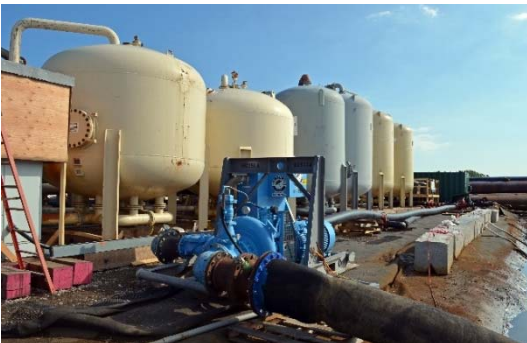
Figure 7: Water treatment plant
