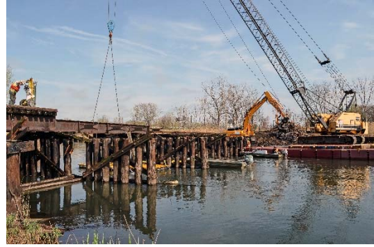
Figure 2: Demolition of the railroad bridge
