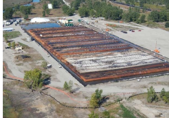
Figure 6: Aerial view of dewatering area
