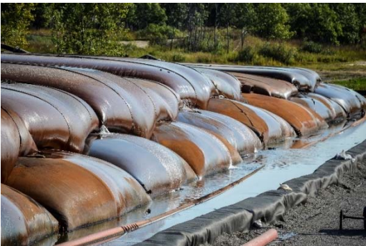
Figure 5: Geotextile dewatering
